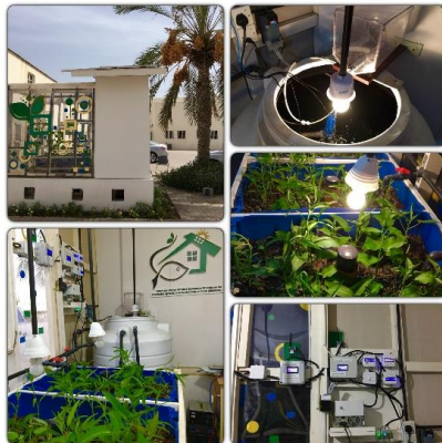
Fig. 2. The actual aquaponics greenhouse facility and the set-up inside it - aquaculture tank, hydroponic beds, control and monitoring system
