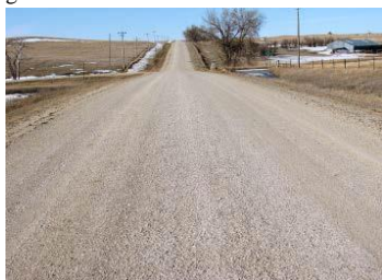
Figure 2: Example of a very good gravel road [1].
