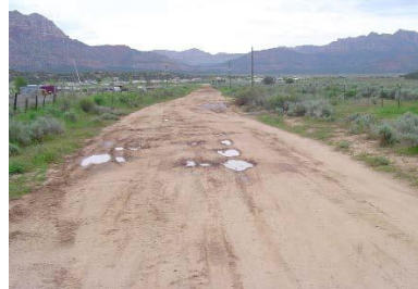
Figure 1: Shows how water contributes to gravel road deterioration [1].
